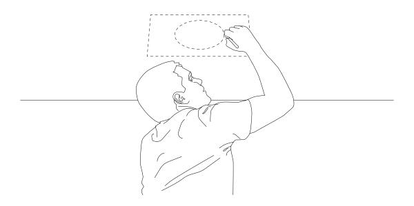
3. Cut around the marked area and remove the piece of drywall.
